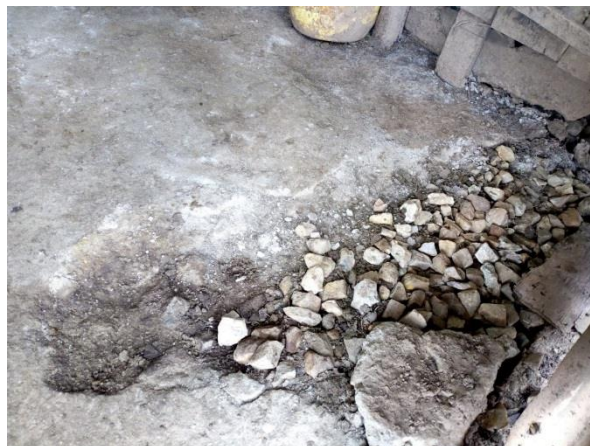
Plate 5.5 Rough broken floor in Shibuli ward, Kakamega central sub county, Kakamega County, Kenya
