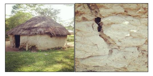
Figure 0:3: A mud hut and crack on the walls
