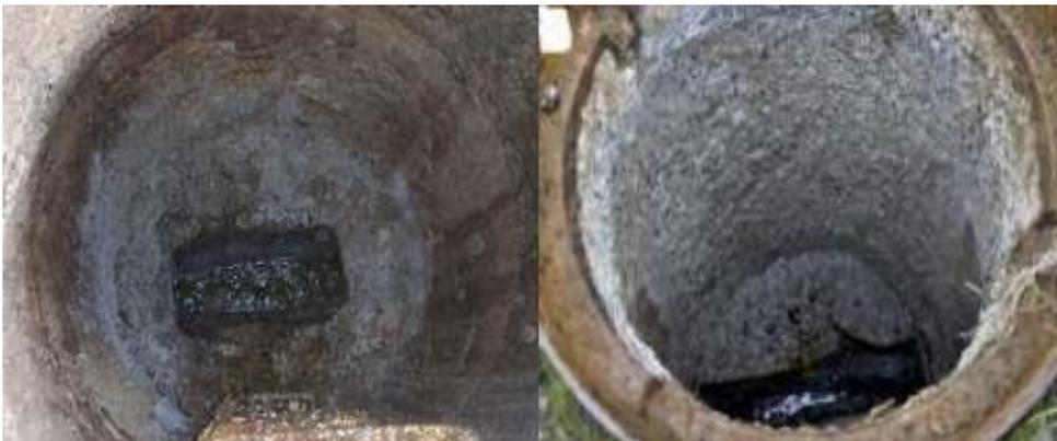
**Figure 1. 5: Internally Corroded Concrete manholes (Guangming, 2014)**
