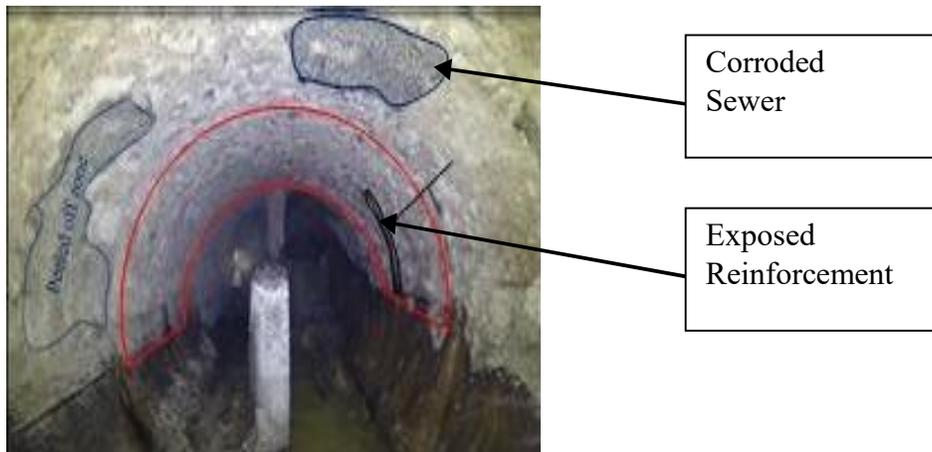
**Figure 1. 2: Corrosion conditions in a sewer tunnel (Limping et al, 2018)**
