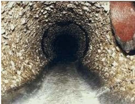
**Figure 1. 4: Internally Corroded Concrete Sewer Pipe (Guangming, 2014)**
