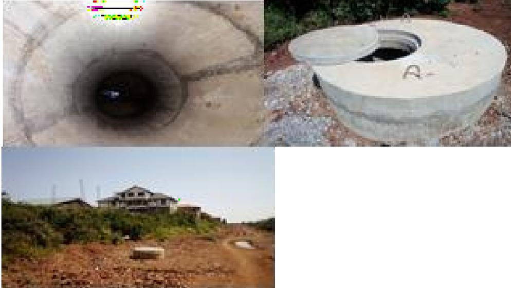
**Figure 1. 1: Newly Constructed Concrete Sewer Pipe and Manholes**
