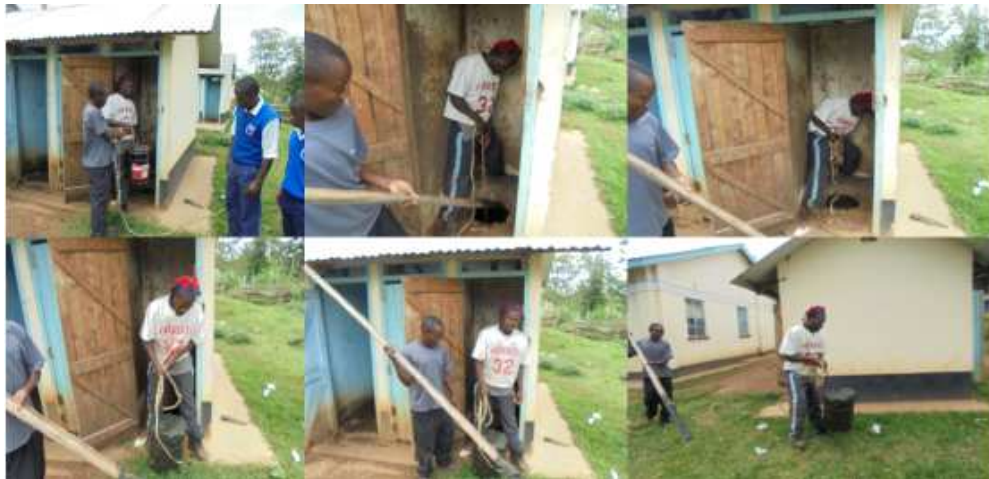
Plate 6: Manual method of emptying filled up pit latrines in some schools
