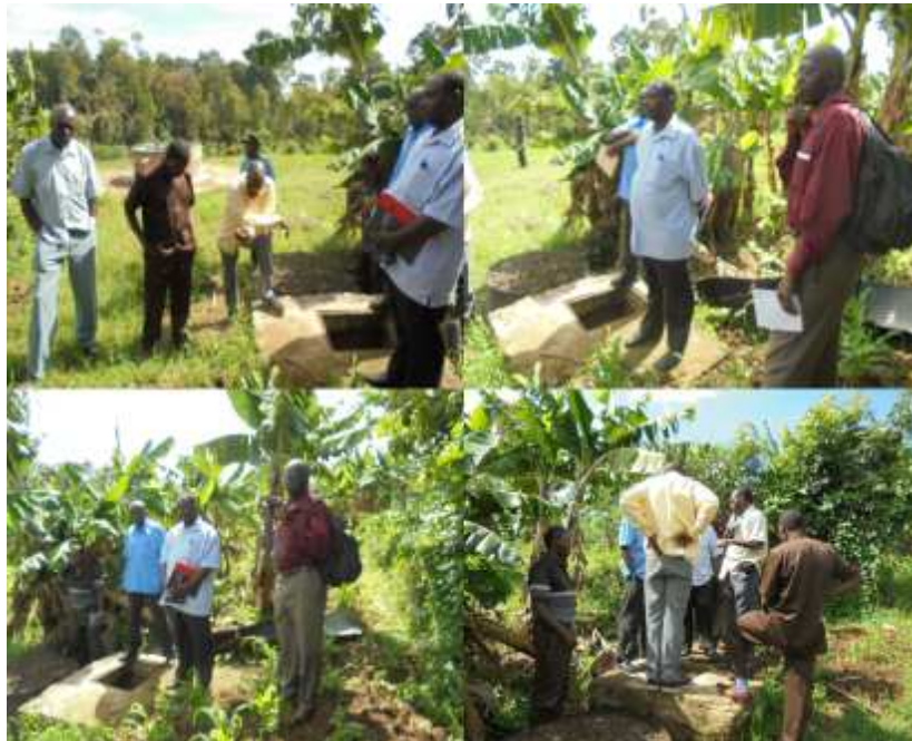
Plate 16: Researcher Supervisor & Engineers at the Kaimosi TTC sewage biogas plant
