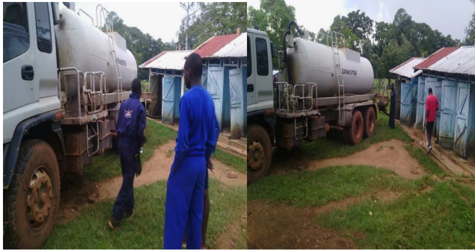
Plate 5: Mechanical method of emptying filled up pit latrines in some schools
