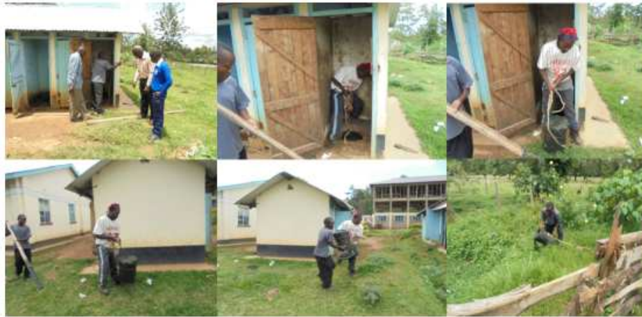
Plate 7: Manual method of emptying filled up pit latrines & disposal
