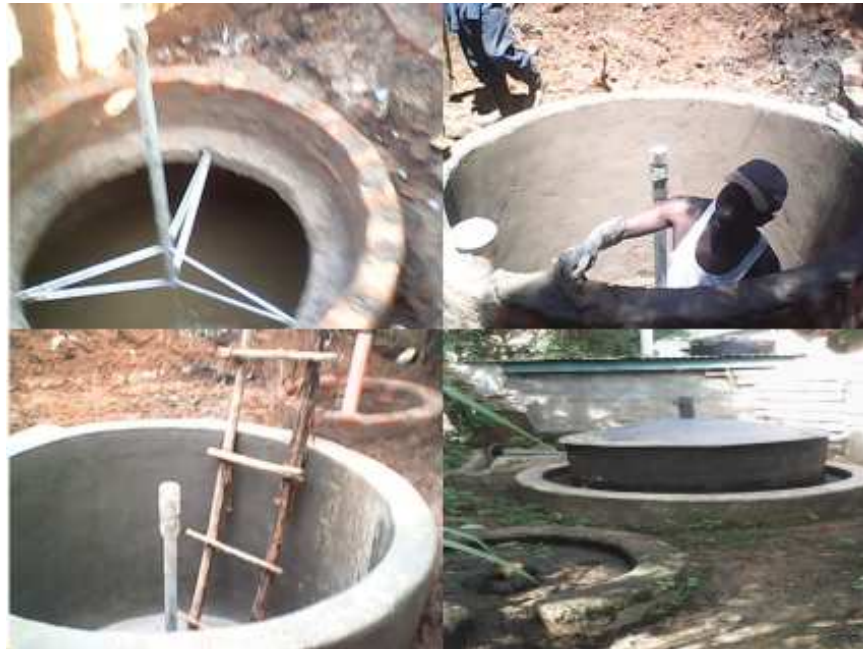
Plate 12: 10m 3 Biogas Digester Plant under construction and a functional one
