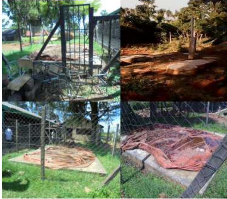
Plate 19: Biogas collecting point
