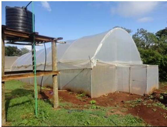
Fig. 4: A properly set high tunnel with double exclusion door, foot bath, insect proof net and roll ups
