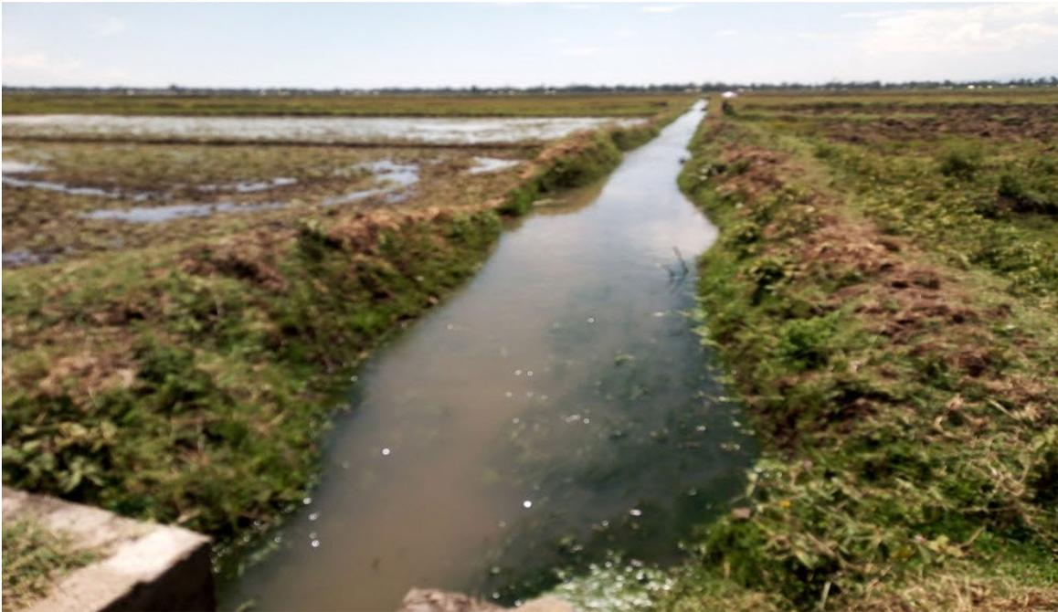
Figure 4 Canal network with excessive underbrush and weeds.
