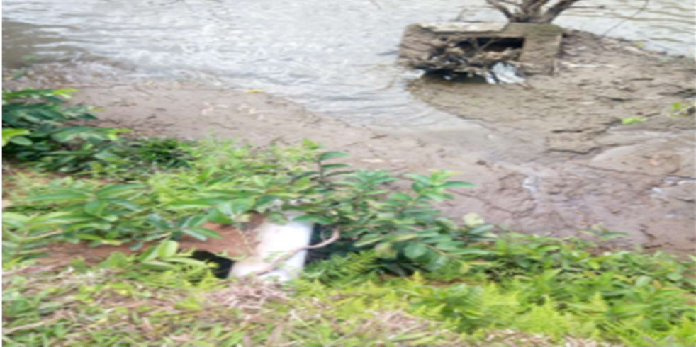
Figure 6: Broken down effluent pipe in River isiukhu
