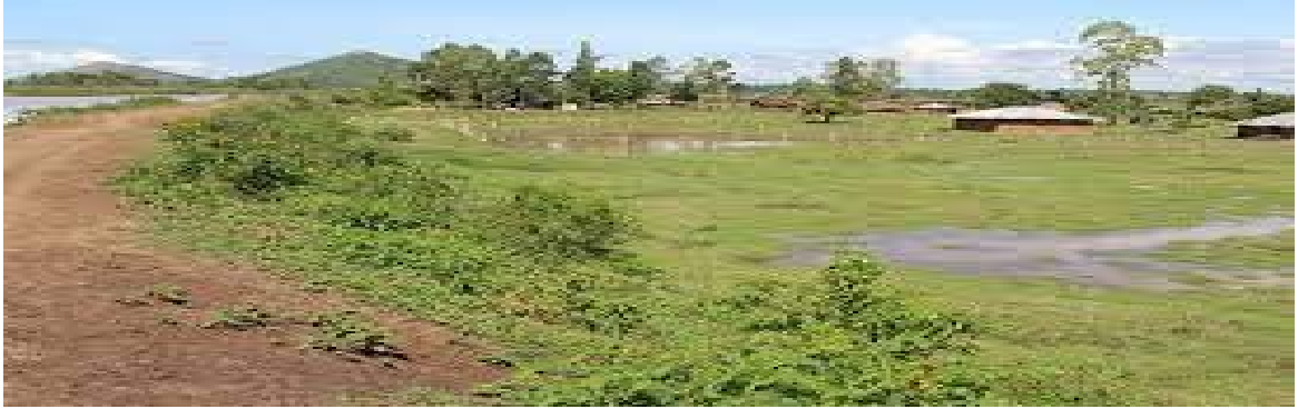
Plate 5.10: Part of the earth dyke for flood management in Nyadorera in Alego Usonga Sub County
