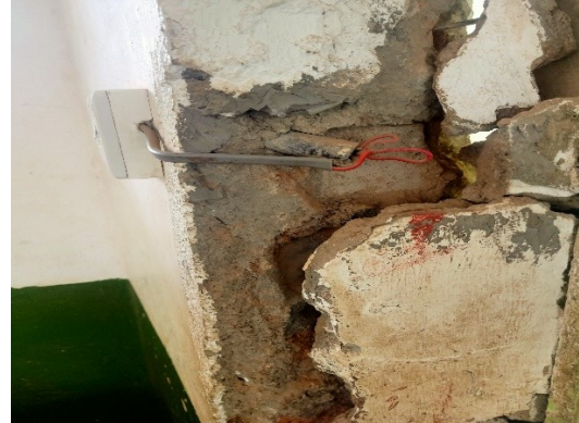
Plate 5.2: Electrical switch in a class
